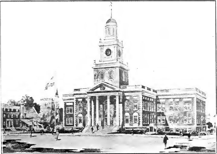
NEW MUNICIPAL BUILDING
